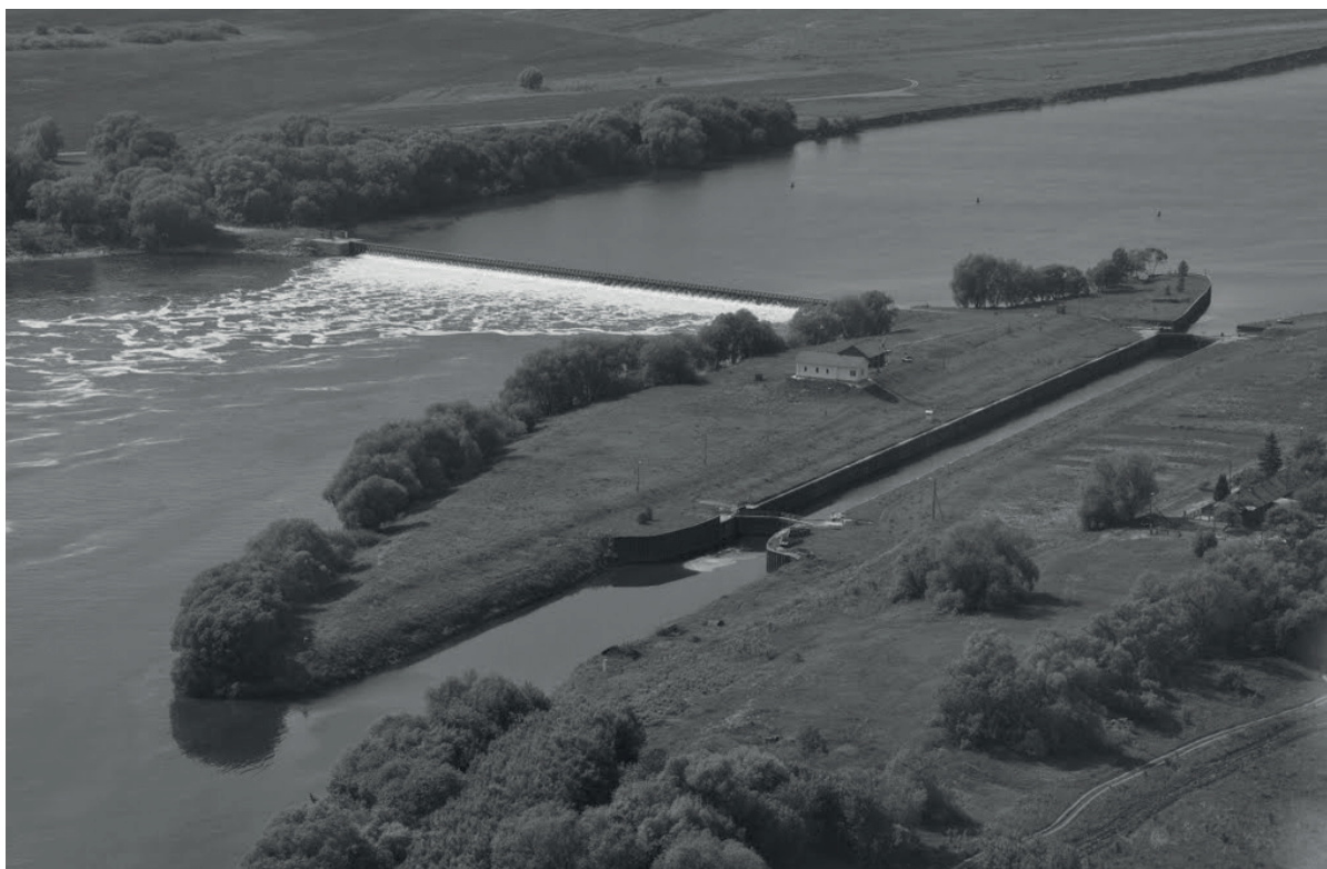
Figure 2. Beloomut lock and dam
